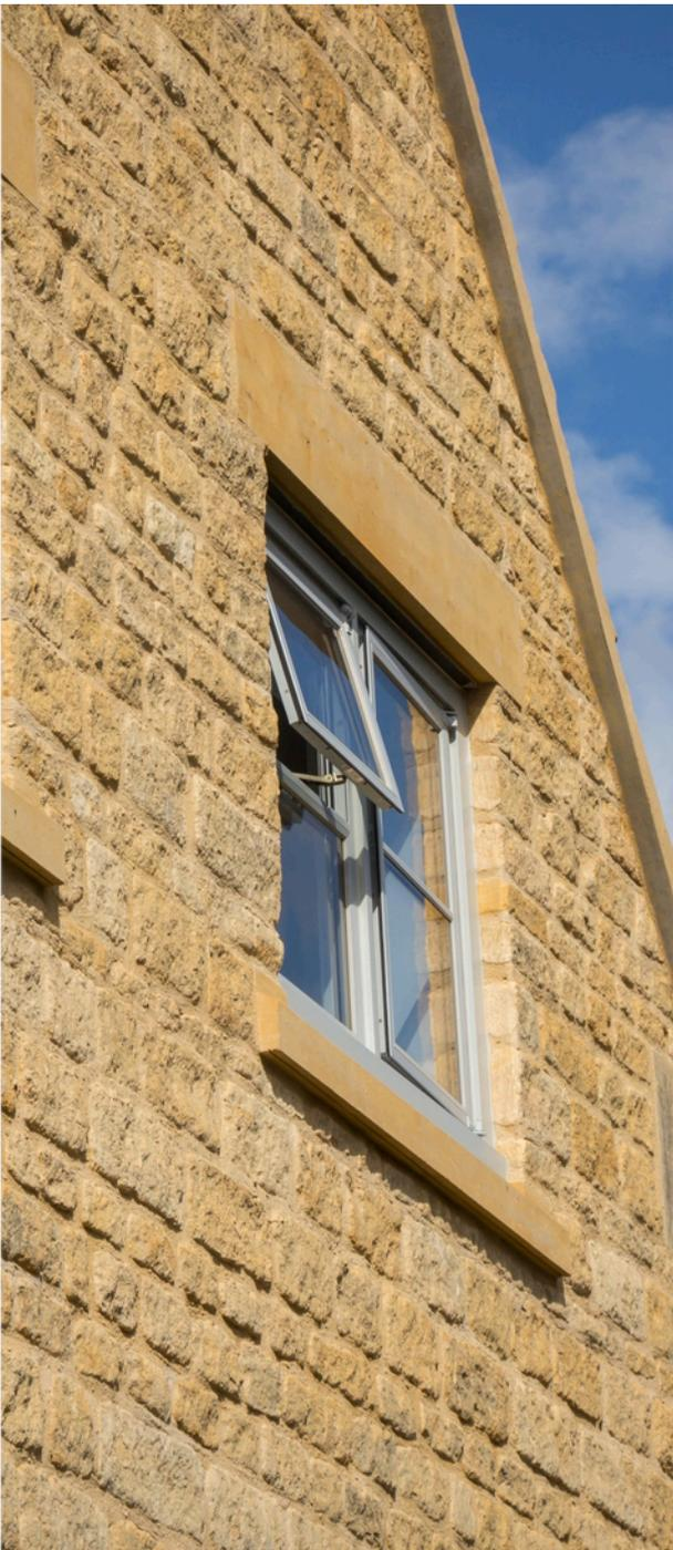
There are many different materials of choice when specifying window and door frames; however steel has long been recognised as a secure material, due to its inherent strength, which makes steel framed windows and doors difficult to force open by the opportunist thief.
